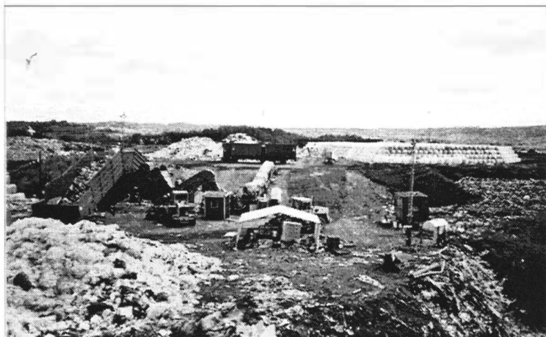
GRAAB recovery station at Tagene, Gothenburg with a storage of 28 000 bales 1997.
