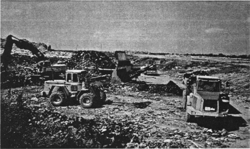
Photograph 1. Excavator, front loader, dumper and drum screen used during excavation.
