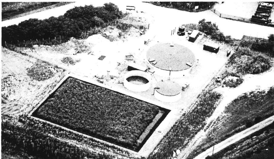
Figure 2. Efford Leachate Treatment Plant, from the North, 10 July 2003.
