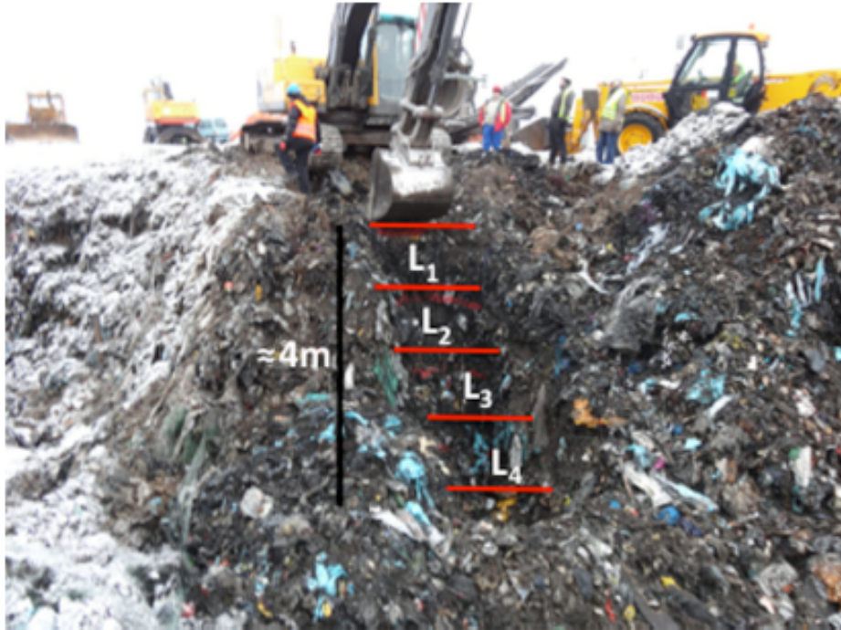
Figure 1: Excavation of test pit 1 (TP 1 ) with excavation layers indicated in red lines
