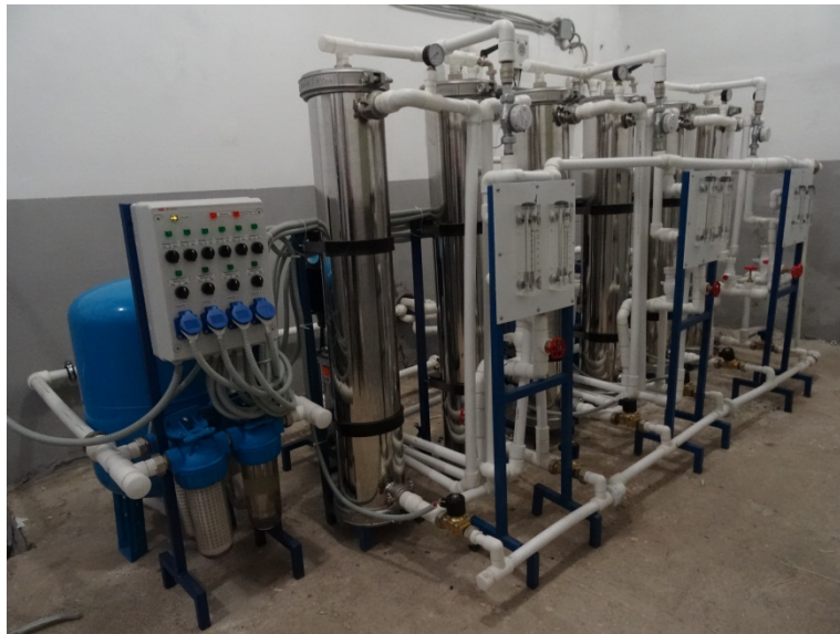
Figure 8. Double stage RO membrane unit for wastewater treatment, 6,5 cubic meter per hour capacity: operation of the membrane unit at local storm water treatment facilities (FSUE TSENKI, Moscow, Russia).
