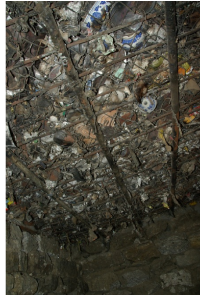
Figure 2. Top pictures shows advanced incinerator in Lukla, today it is used just as an open pit incinerator as parts for maintains don't exist. Bottom pictures shows a well design open pit incinerator in Namche that could work very well for its purpose but because of insufficient sorting it is filled up with non-burnable waste.
