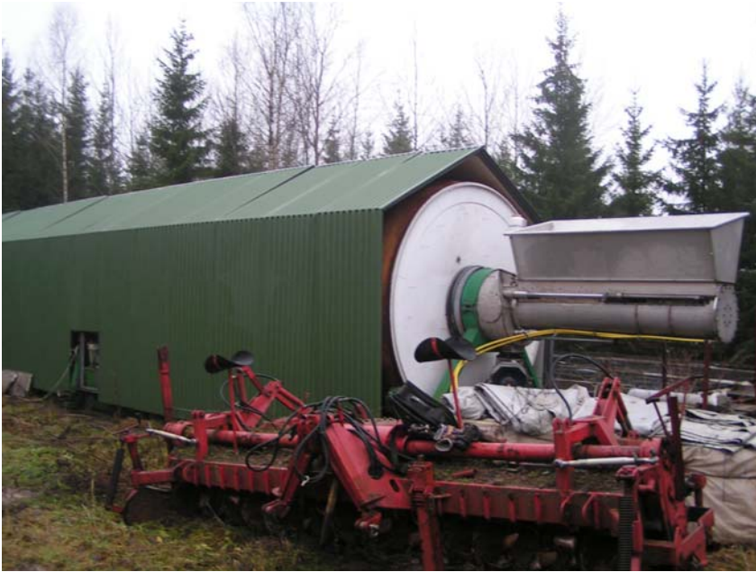
Figure 2. The solid phase reactor for biogas production from lay crops outside Sala.
