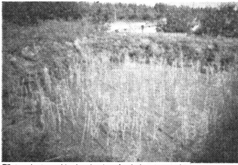
Pilot project: reed bed technology in sludge dewatering
