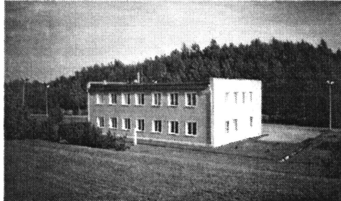
Main building of Põlva Wastewater Treatment Plant
