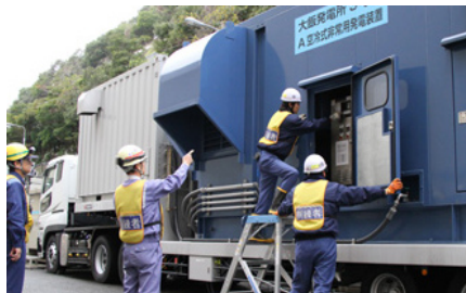
Installation of Redundant and Diversified Power Supply
